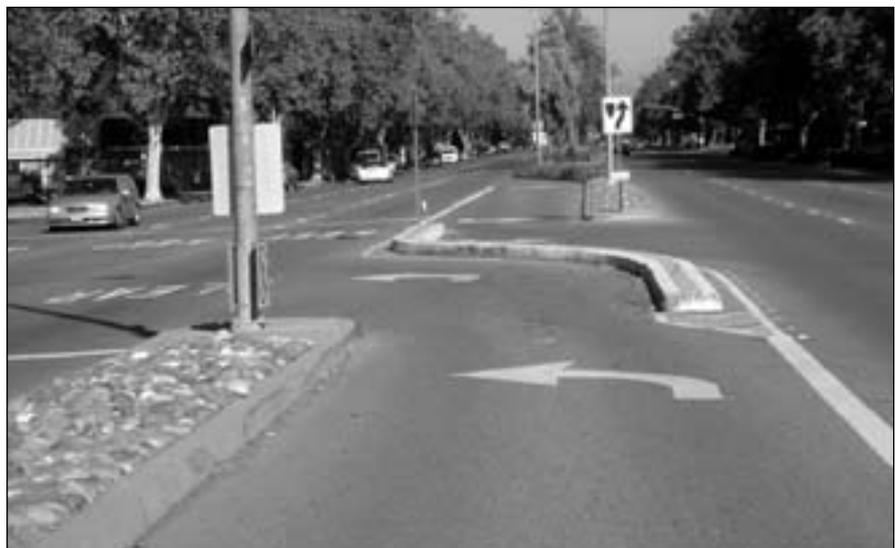
**Figure 3.** The full median opening was converted to a directional opening because of the numerous collisions involving crossing maneuvers and left-turns onto the major roadway. Location: Santa Rita Road, Pleasanton, California
